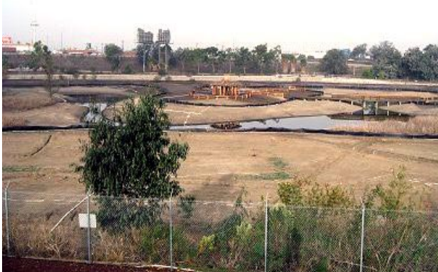
Construction and enhancement of the marshland took two years to complete.
