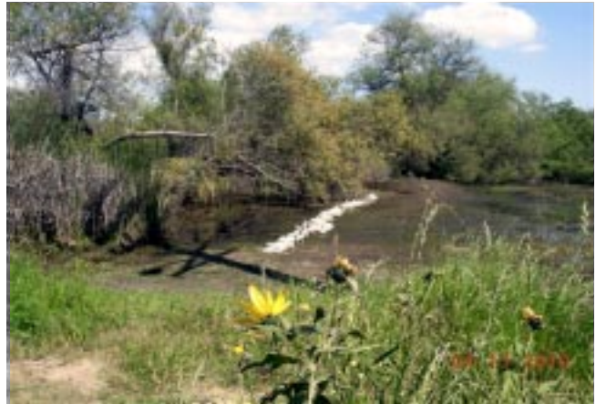
Sandbags are placed to hold water in northwest Marsh.
