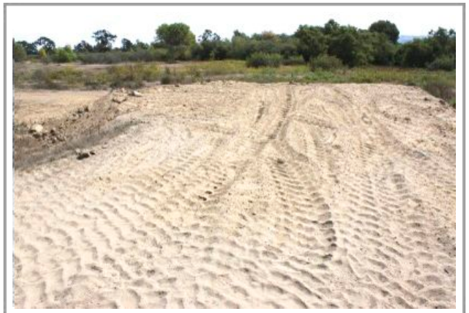
Newly added portion of Observation Berm, taken from top of berm.
